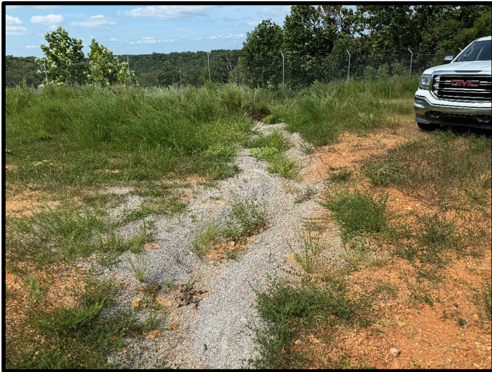
Photograph 14: View of washout present in road between LCS-4 and LCS-5.
