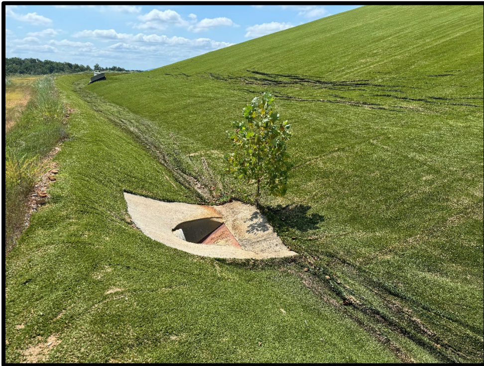
Photograph 16: View of woody vegetation growing in closure turf near LCS-7.
