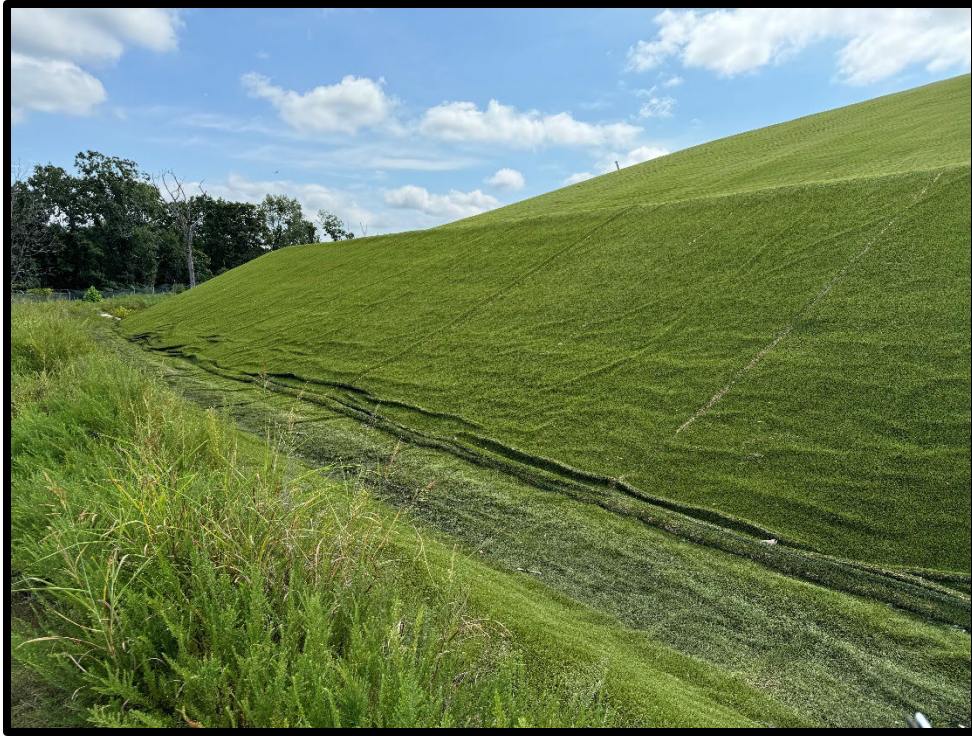
Photograph 9: View of rills present in closure turf of north side of Area 1-2.
