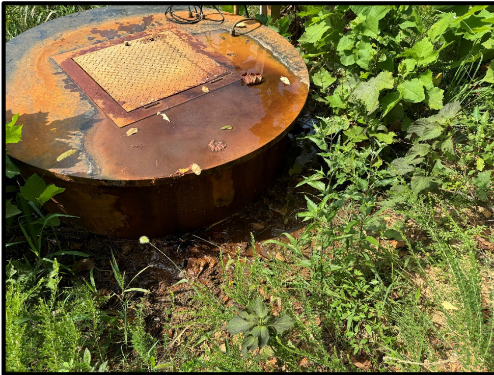
Photograph 2: View of VLCS-1 overflowing to ground.
