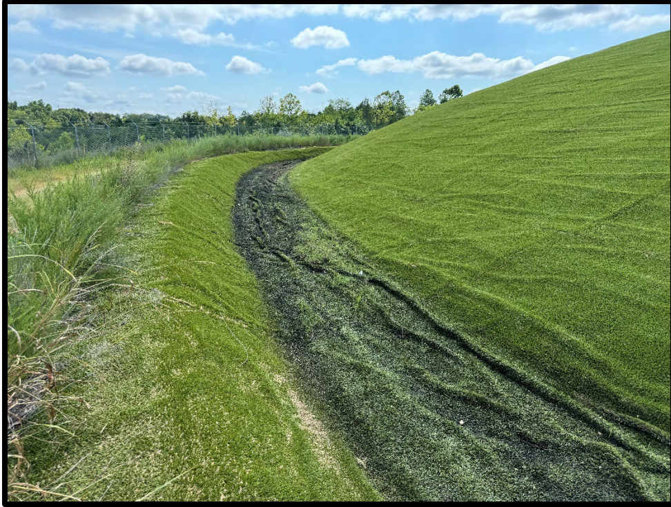
Photograph 5: View of rills present in closure turf of north side of Area 1-2.
