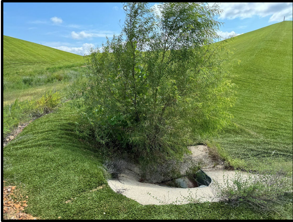
Photograph 15: View of woody vegetation growing in closure turf near LCS-5.
