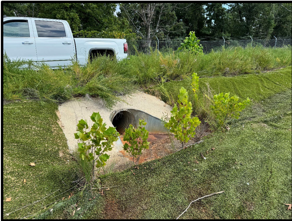
Photograph 8: View of woody vegetation growing in closure turf on north side of Area 1-2.
