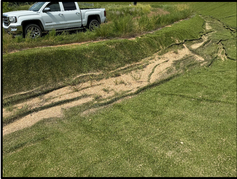
Photograph 13: View of sediment present on closure turf near LCS-4.
